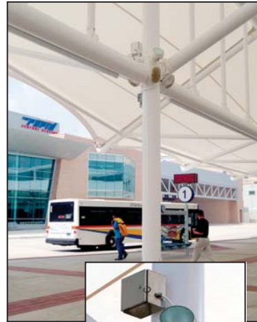
The external speakers on the transfer platform are mounted on the column.
