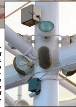
The external speakers on the transfer platform are mounted on the column.
